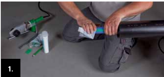
Remove dirt and impurities at the pipe ends. (Note: for the processing of aquatherm blue pipe of ti, also see description on page 22)
