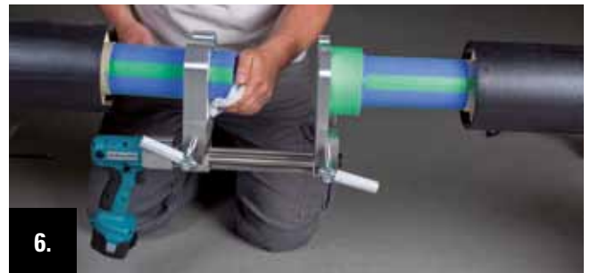
6. Remove dirt and impurities from the pipe end and from the inside of the fitting.
