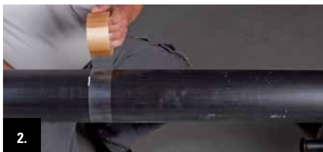
2. Mark the cutting line with an adhesive tape around the pipe.
