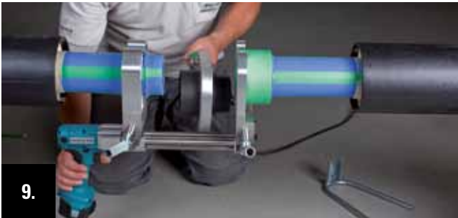
9. After the end of the heating period drive the welding jig apart and remove the welding device between pipe end and fitting.
