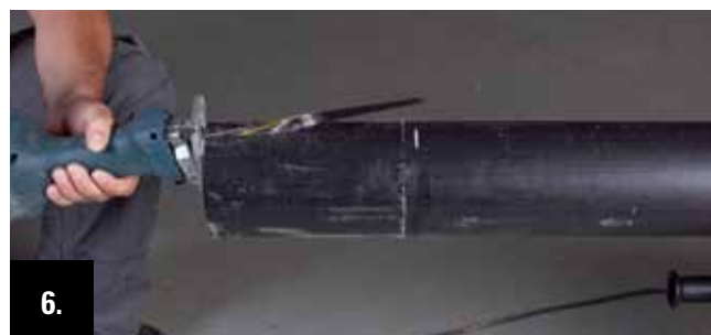
6. Slit the casing up to the PUR-insulation layer with a customary handsaw for plastic.
