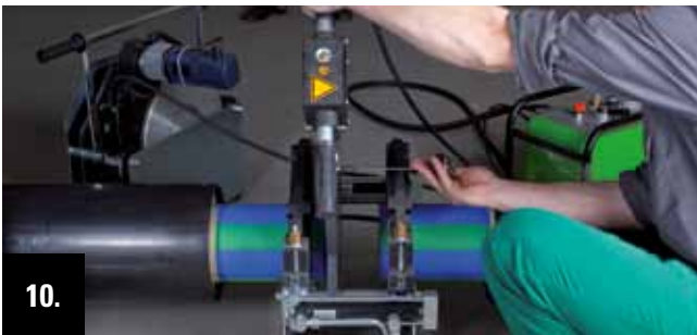
10. Insert the welding device between the pipe ends. Check, if the welding plate is clean and measure the welding temperature.
