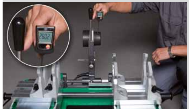
Measurement of temperature at the aquatherm- welding machine
