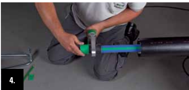
Press the aquatherm-socket on the male welding tool and at the same time push the pipe end up to the marked welding depth in the female welding tool.
