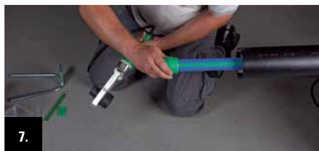
Within the processing time press the welding socket on the pipe end up to the end of the welding depth.
